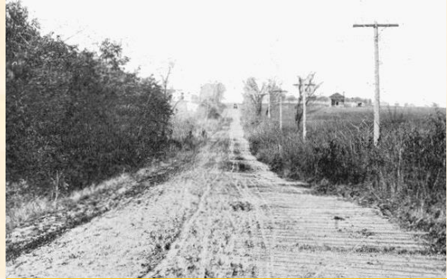
This plank road near Belleville, Ill., is planked on the right side only.
